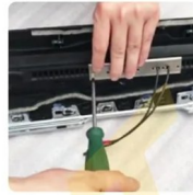
6. Fixed mounting iron plate
